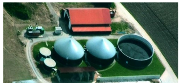
Fig. 4 Technological buildings of biogas station [6]
